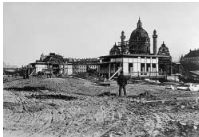
The station in Karlsplatz under construction
