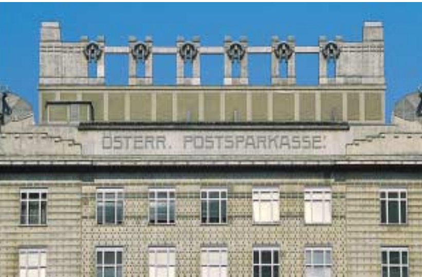
Otto Wagner, façade of the Postal Savings Bank
