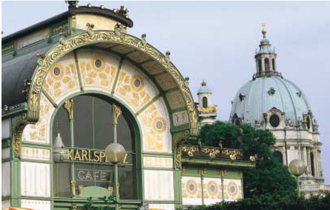
Otto Wagner's station in Karlsplatz today
