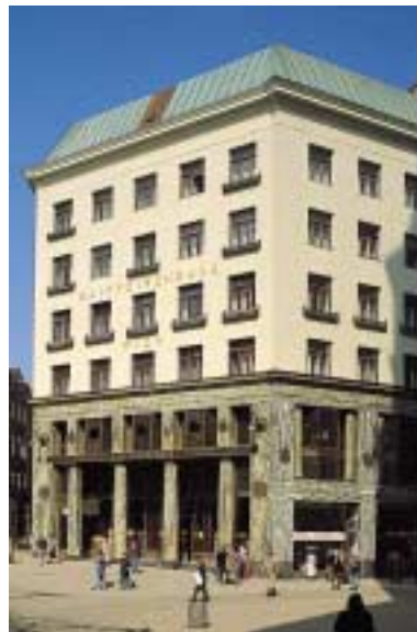
The house built by Adolf Loos for Goldman & Salatsch in Michaelerplatz
